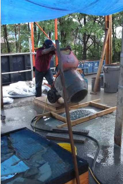
Above left: Existing tiles soaking in water in order to facilitate the removal of the tiles from the substrate; above right: soaked tiles are placed in a tumbler to remove the substrate from the tiles; below left to right: tiles in the tumbler; cleaned and polished tiles are mixed with new tiles (in order to compensate for loss) and placed in plastic bags; cleaned tiles are removed from the tumbler and placed on screens
