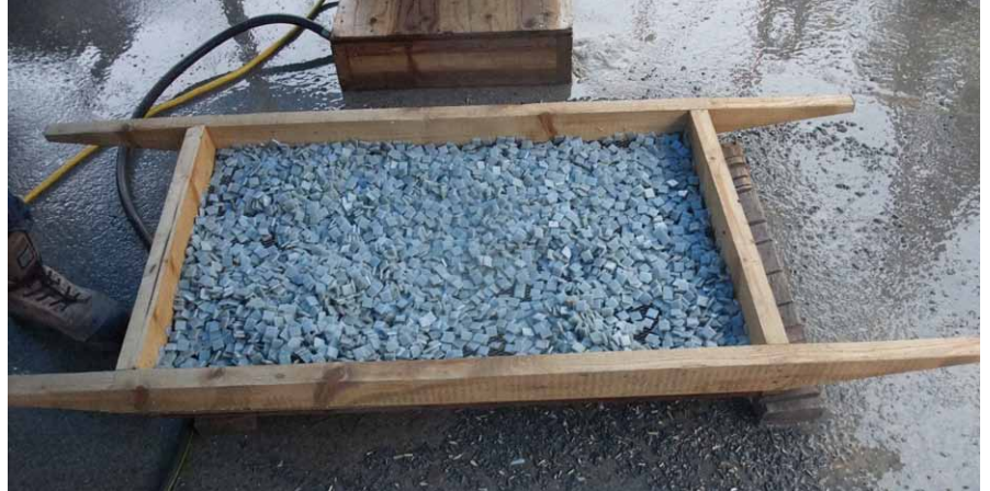
Above left: Existing tiles soaking in water in order to facilitate the removal of the tiles from the substrate; above right: soaked tiles are placed in a tumbler to remove the substrate from the tiles; below left to right: tiles in the tumbler; cleaned and polished tiles are mixed with new tiles (in order to compensate for loss) and placed in plastic bags; cleaned tiles are removed from the tumbler and placed on screens
