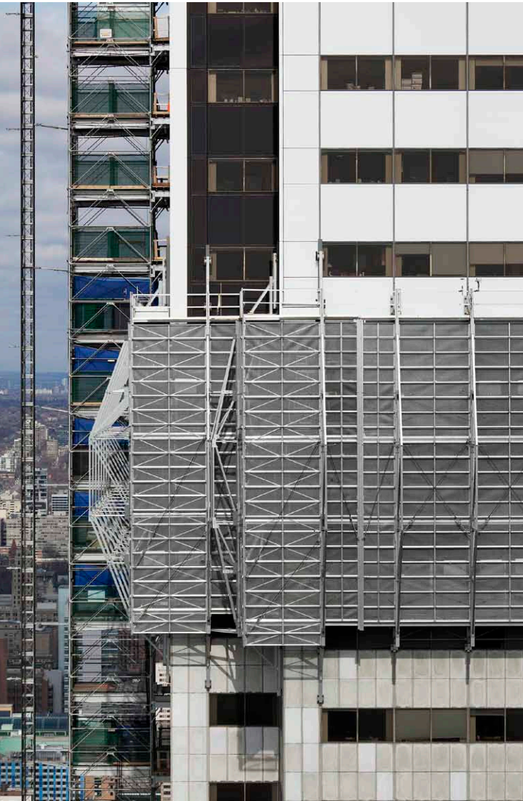
View of moveable scaffolding system (photo credit: Tom Arban).
