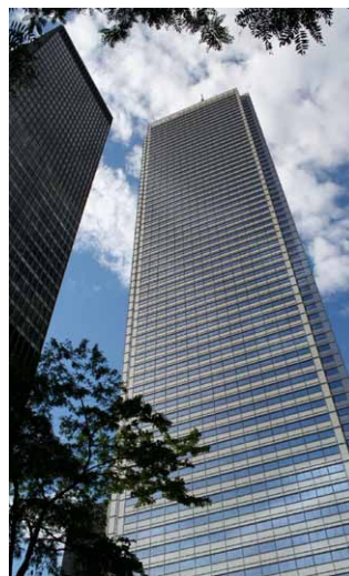
Full Re-Clad Glass spandrels, aluminium sunshades
