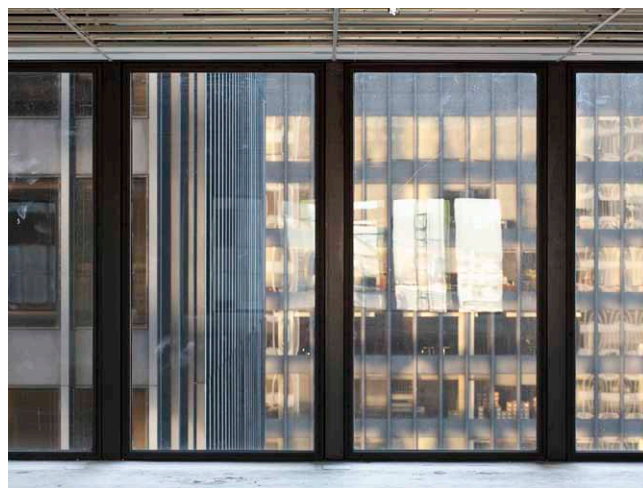
Above left: window - before revitalization (with induction units); above right: window - after revitalization (without induction units).
