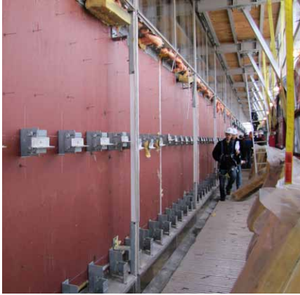
Level 1: Stone removal and remediation deck (Photo credit: B+H)
