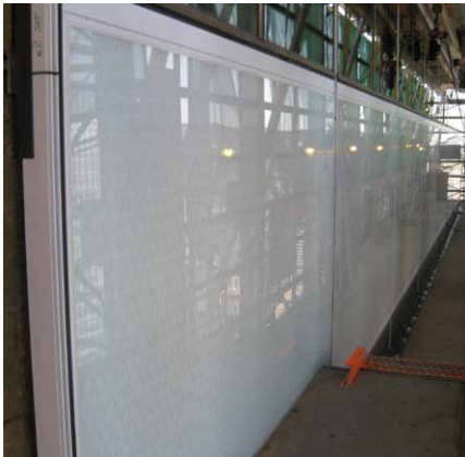
Level 3: Curtainwall installation deck (Photo credit: B+H)
