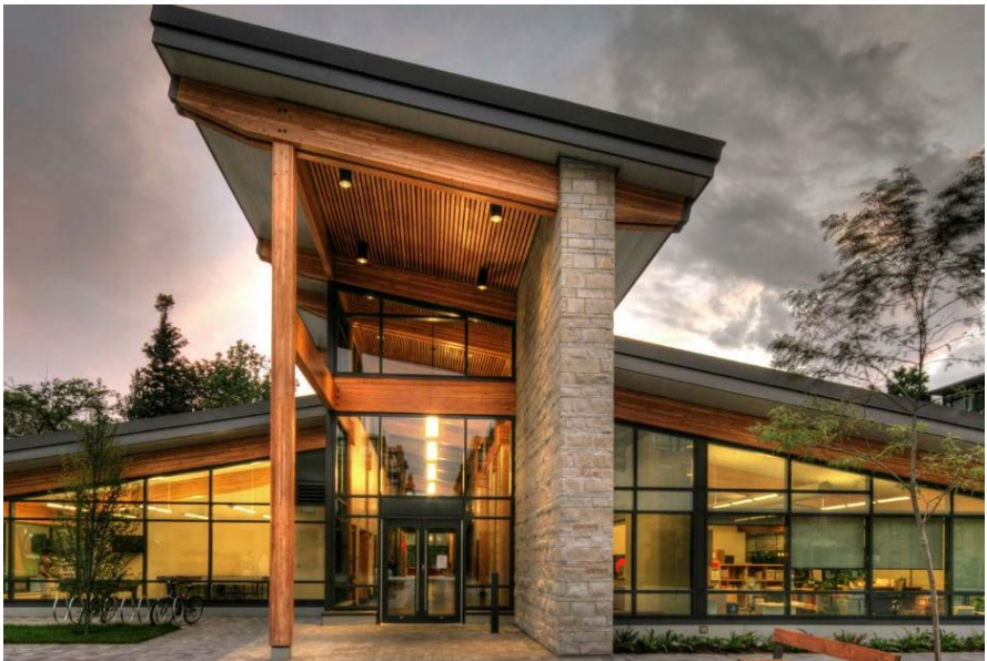
Caption: UBC Marine Drive Amenity Building: Glulam columns and beams support CLT roof panels.
